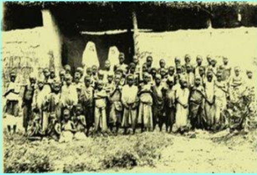
Outside first classroom building at Nsambya
